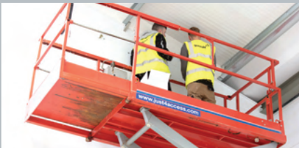
Firestopping installed by our accredited installers
