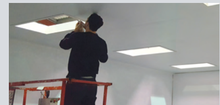
Seal joints where required
